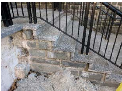
Failing masonry work at exterior stairs
