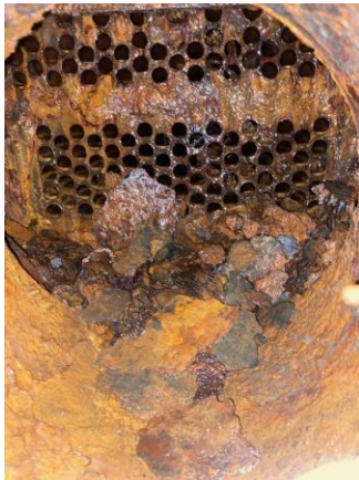
Old condensate pipes scaling
